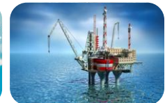
Oil & gas recovery
